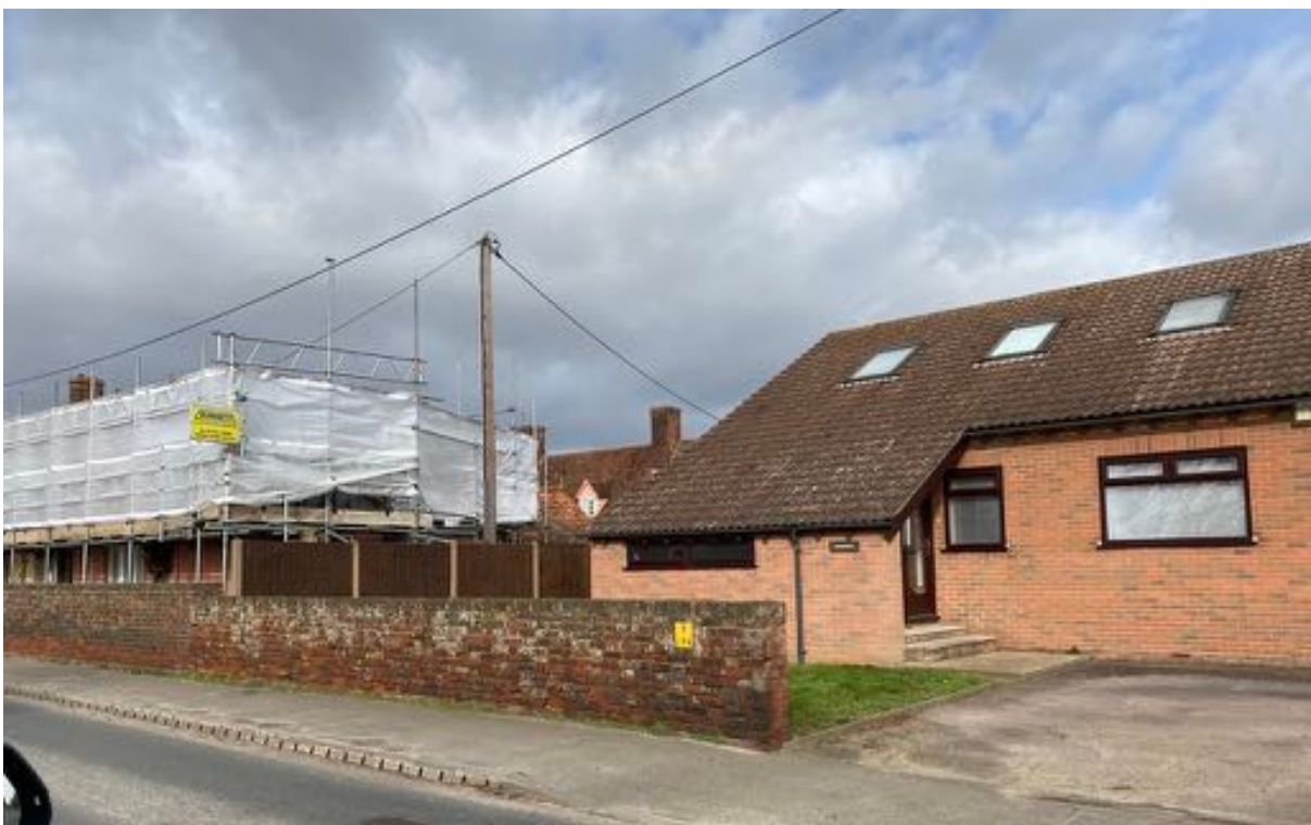
'Shed roof' on A134
