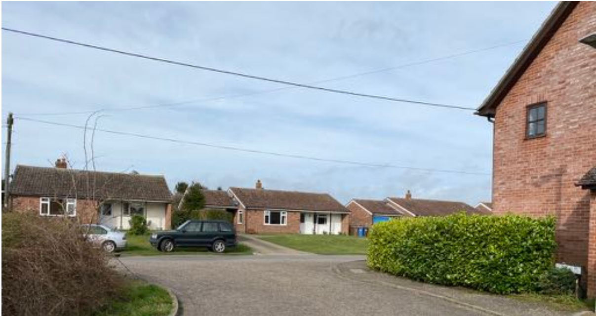
20 th century bungalows off Church Road, from Nicholsons Court
