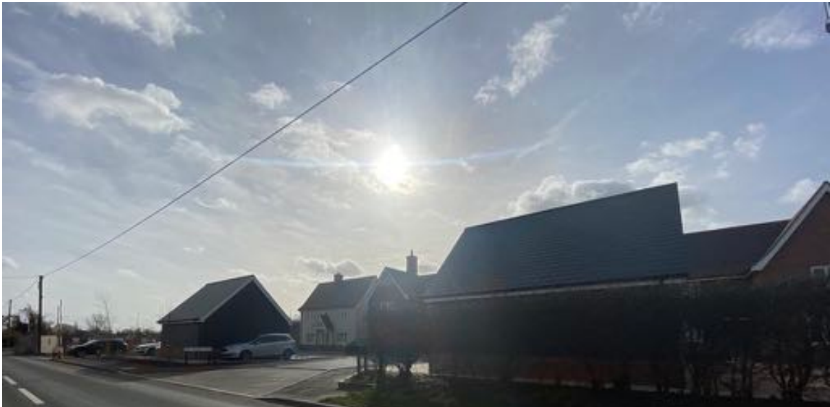
Residential development under construction on A134
