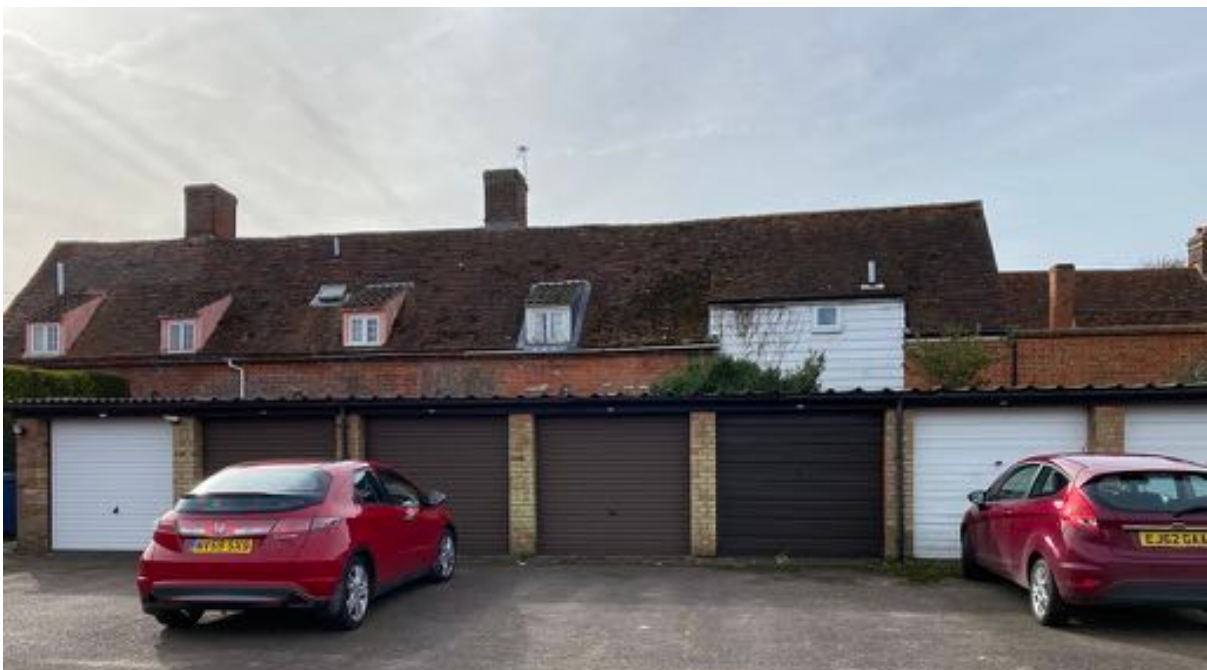
Garages off Plampin Close, in front of historic dwellings
