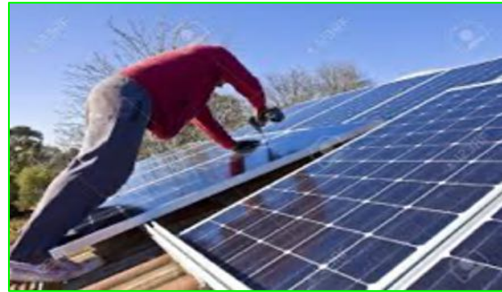
Installing solar panels
