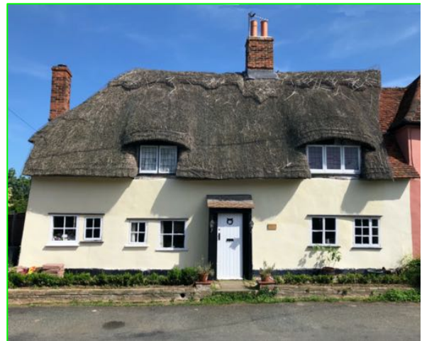
17 th -18 th Century timber frame house
